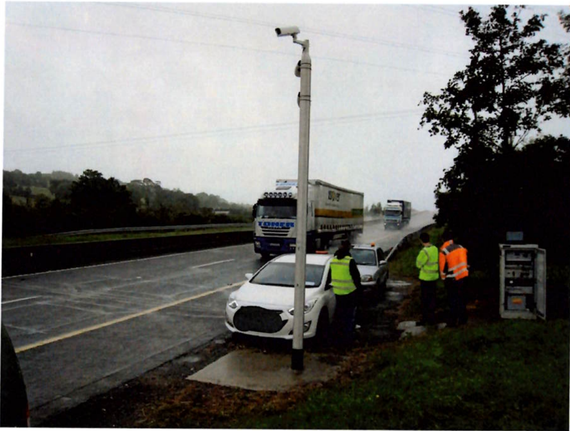
Photo above Weight in Motion Traffic cameras and weigh sensors installed in the road National Roads Authority.
