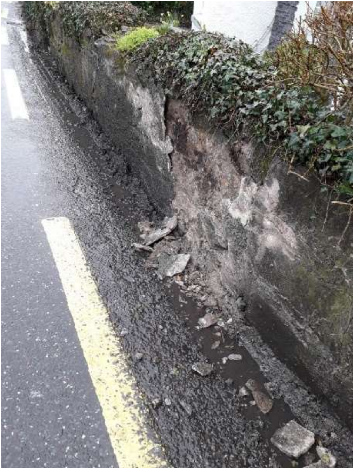
Front wall struck by an HGV 23/01/2019
